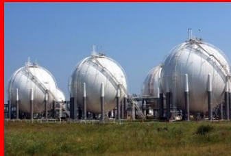
(Petro-)Chemicals & Tank Terminals
